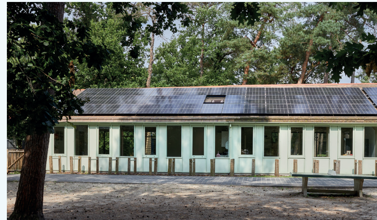
^ Opwek op dak van school in Zeist
