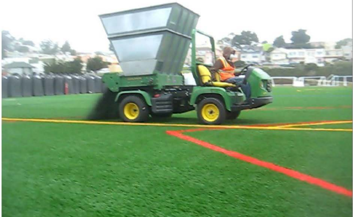
Figure 3.2 Semi-mechanised application of infill
